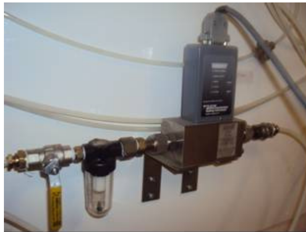
Figure 6-21: Thermal mass flowmeter
