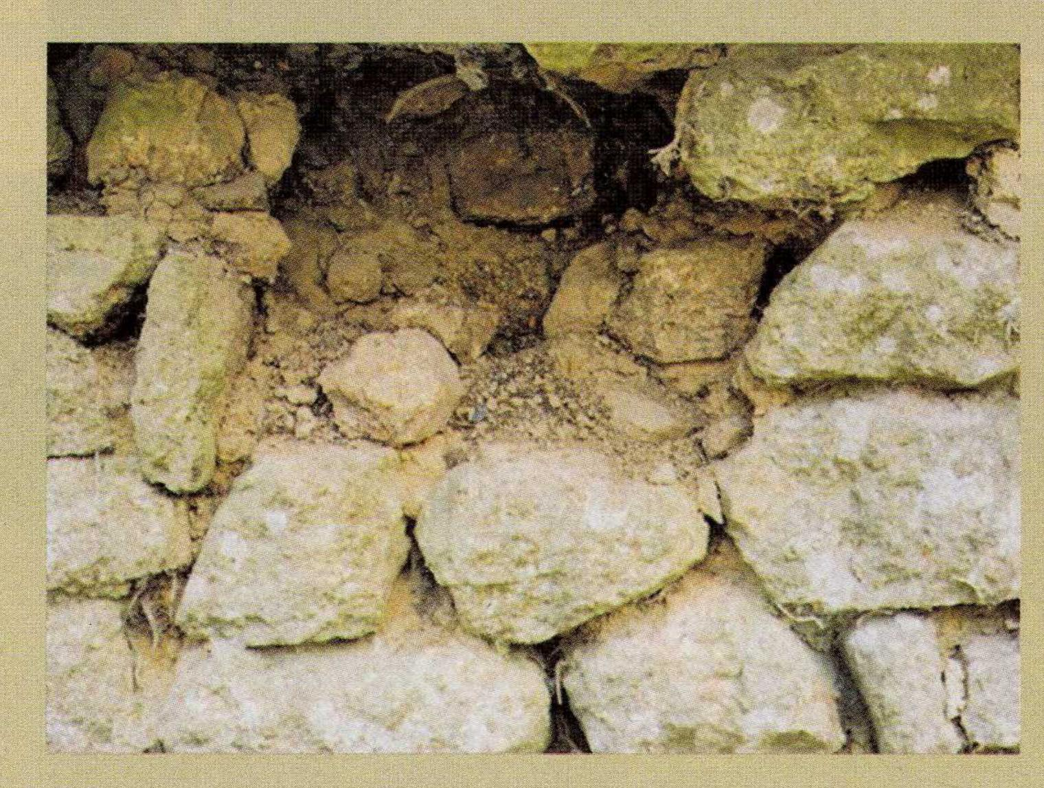
the drying-out of some traditional materials resulting in shrinkage cracks and in some cases structural failure.
