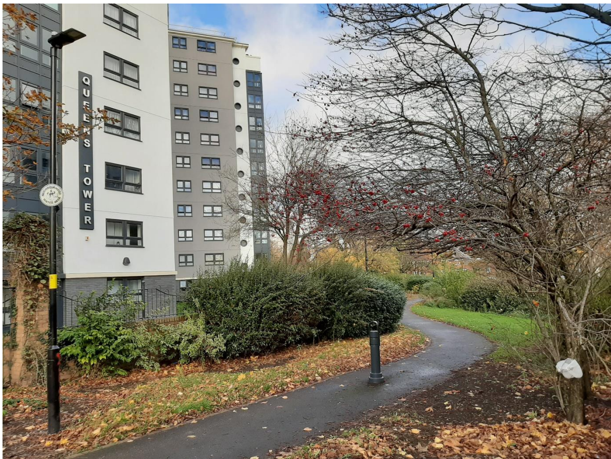
Figure 1: Repeat robbery location: sinuous footpath with poor surveillance opportunities between the recently refurbished Queens and Home Towers at the CSS in 2020
