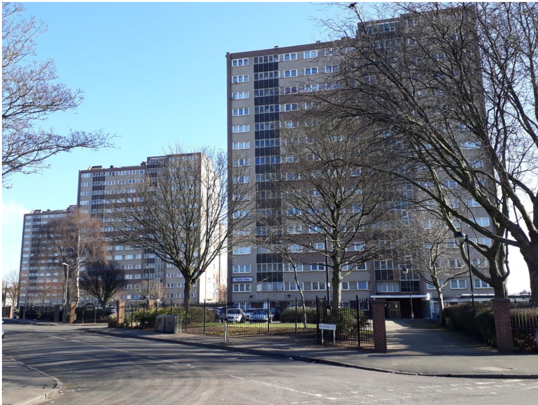
Figure 3: Severn, Medway and Thames Towers – the comparison site in 2017
