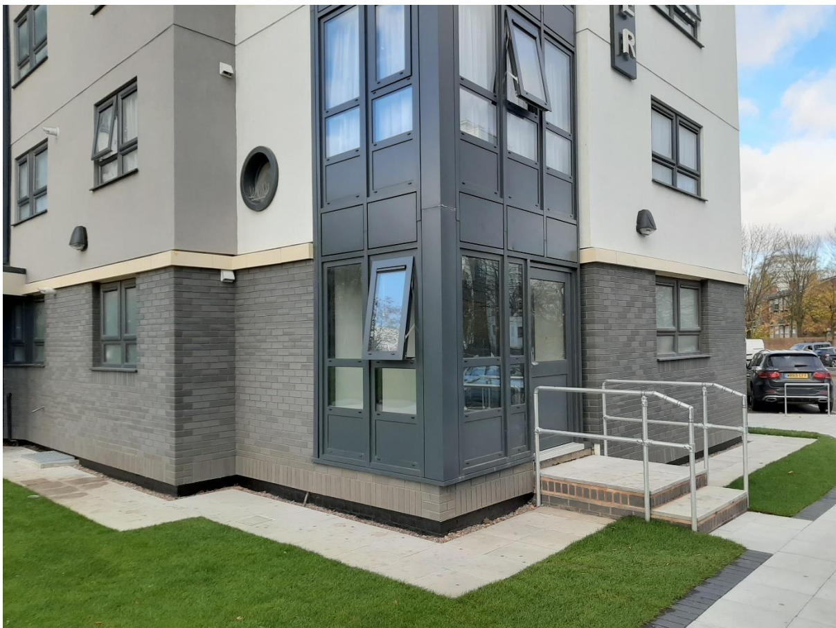
Figure 5: Following the 2018-2020 major refurbishment of the CSS, all the balconies are now enclosed and protected at ground floor level by outward-opening fire-doors. The location of the internal fire-escape staircase is indicated by the round porthole style window.
