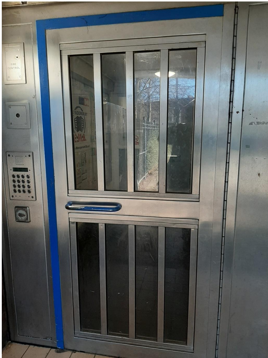
Figure 7: Ground floor communal entrance door at Medway Tower, comparison site, controlled by fob-reader electronically-operated opening system and with both audio and video link to offsite control room.
