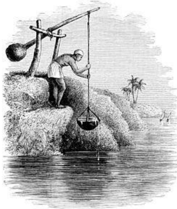
Figure 1- A shaduf device (Mirti, 2001)
