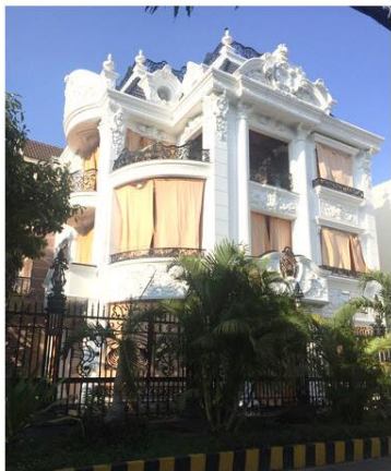
A new 'old-style' villa (Source: Nguyen Thanh Tuan)
