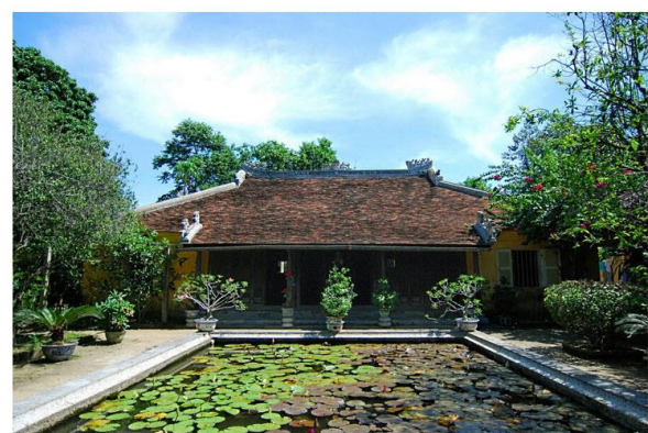
An Hien vernacular house, Hue city (Source: vnexpress.net)
