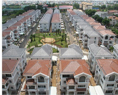
Project in Ho Chi Minh city Land area: 275 m 2 Land coverage: 60% (Source: cuongthinhland.vn)
