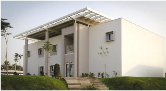
A PH office building in Dubai (2016) (Source: passivehouse-database.org)
