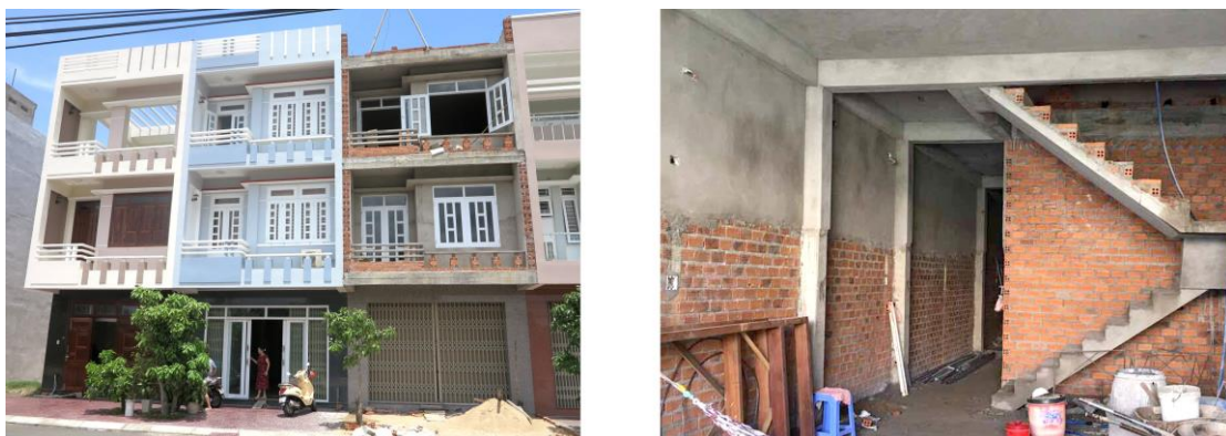
Figure 5.3: Terraced houses in Vietnam
