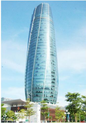
Danang Administration Centre (Source: baogialai.com.vn)
