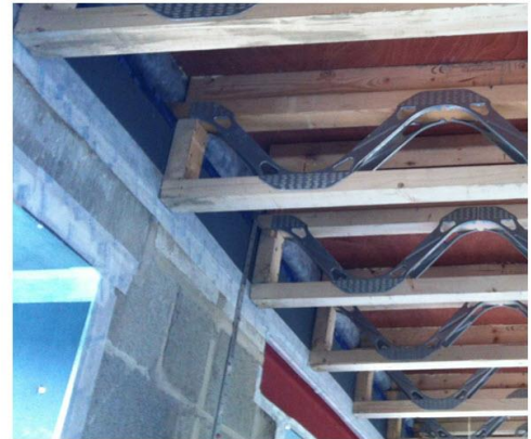
Taping for air tightness in Kirkburton Passive House (Source: author)
