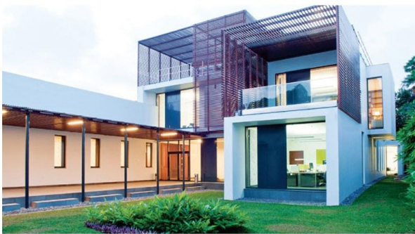
A PH office building in Indonesia (2011) (Source: passivehouse-database.org)
