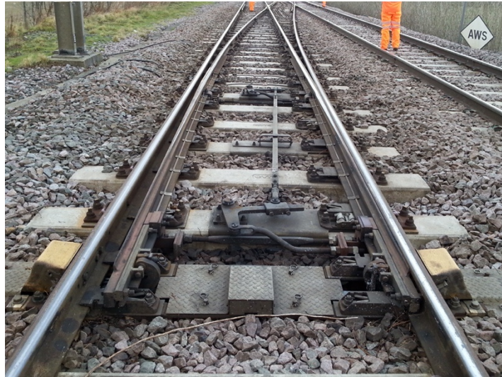
Figure 2.4 – Overview of switch panel including the switch rails and switching machines.
