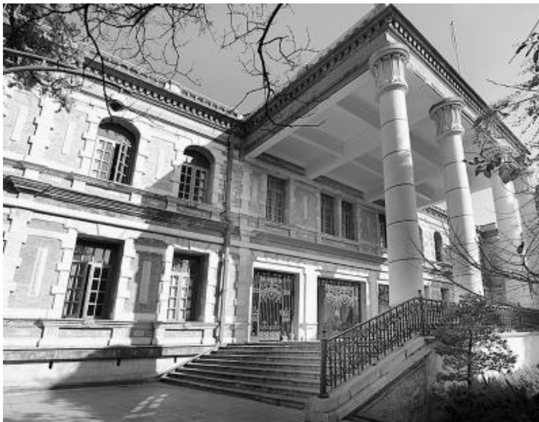
Figure 2.4 Huize Building, location: Yunnan University (Photo by Wen Jiang,2013)
