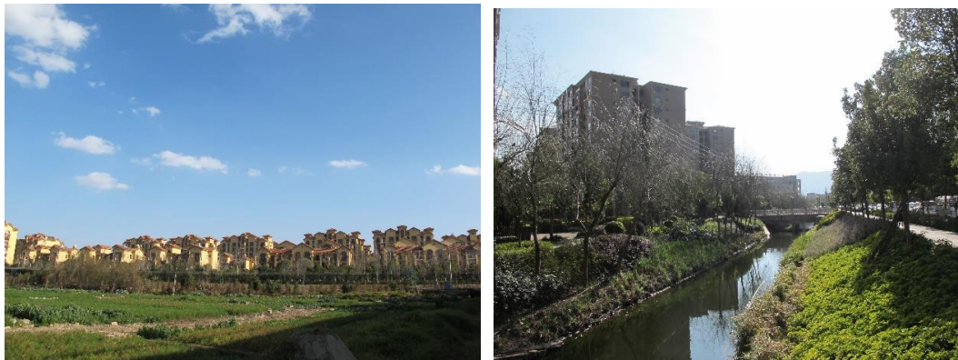
Figure. 5.17 Urban village renovation project, Tai He village, Kunming (Wen Jiang, 2015)
