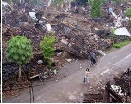
Houses damages from Bantul earthquake
