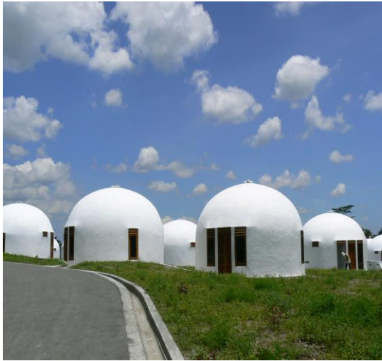
Dome House construction
