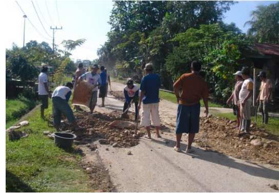
Gotong royong in repairing village road
