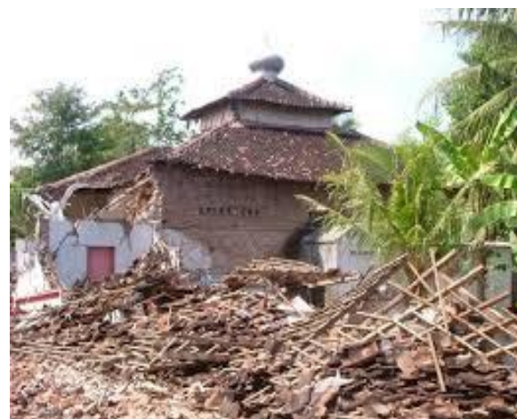
Mosque damages from Sleman earthquake
