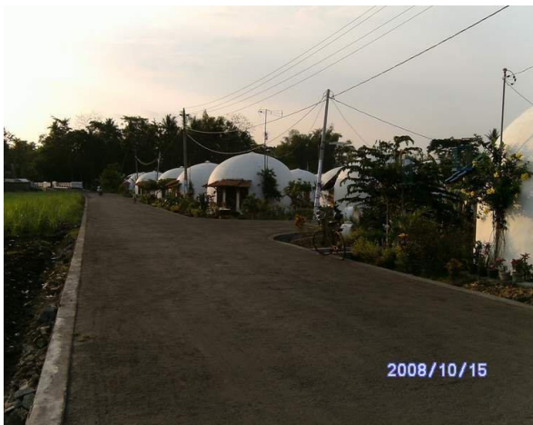
Evacuation road in Ngelepen Dome House
