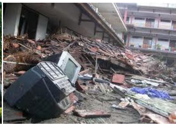
School building damages from Bantul earthquake
