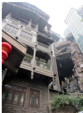
Figure 4. Hongya Dong shopping center in Chongqing, photo by Guo Chen.
