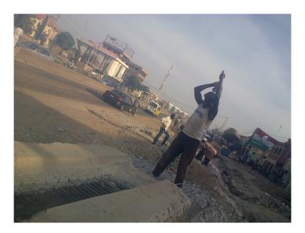
Figure 33: Self-employed *Dangwangwan* breaking concrete to salvage reinforcements for sale
