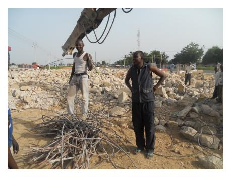
Figure 34: Salvaged reinforcements from a broken concrete
