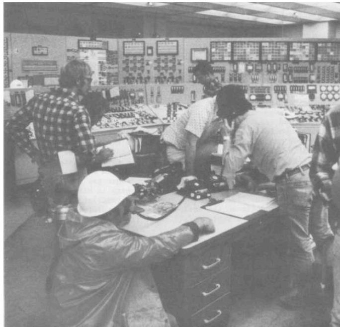
Figure 1: Control room TMI-2 during the accident (Kemeny, 1979)
