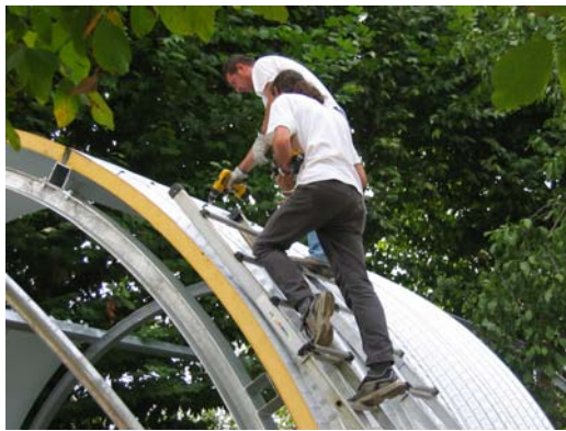
Figures 5,6,7,8 The 3 hinged main arches are in ordinary steel profiles HEA 120 mm and they carry the secondary rectangular beam section profiles on which is fixed the curved Elycop panel. On the floor a sandwich panel of 80 mm which acts as bearing structure fixed on main steel beams. The final shape allows energy equipment to be integrated.
