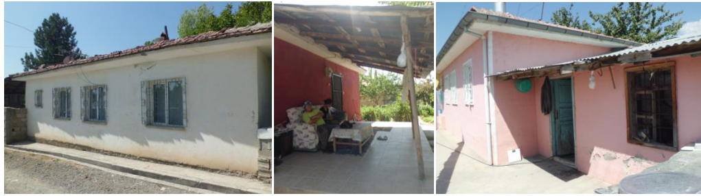
Figure 4 The exterior picture of a maintained house with a facade painted and plastic window profiles; a dweller added a porch to the entrance of the house; another dweller added an extra space to the next of the house (D G Yilmaz 2013).
