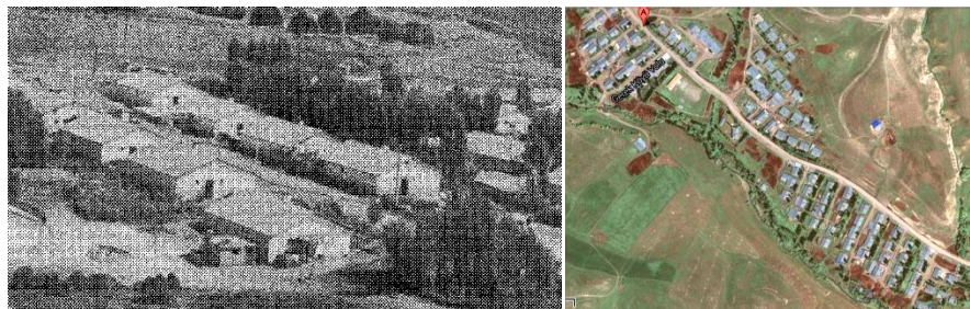
Figure 5 A picture from the implementation for the village, which was totally relocated after the earthquake (Gok 2001); the aerial view of the village today (GoogleMaps 2013).
