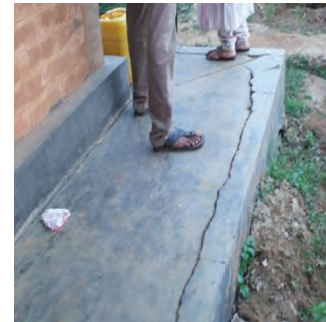
Figure 3 Foundation cracked
