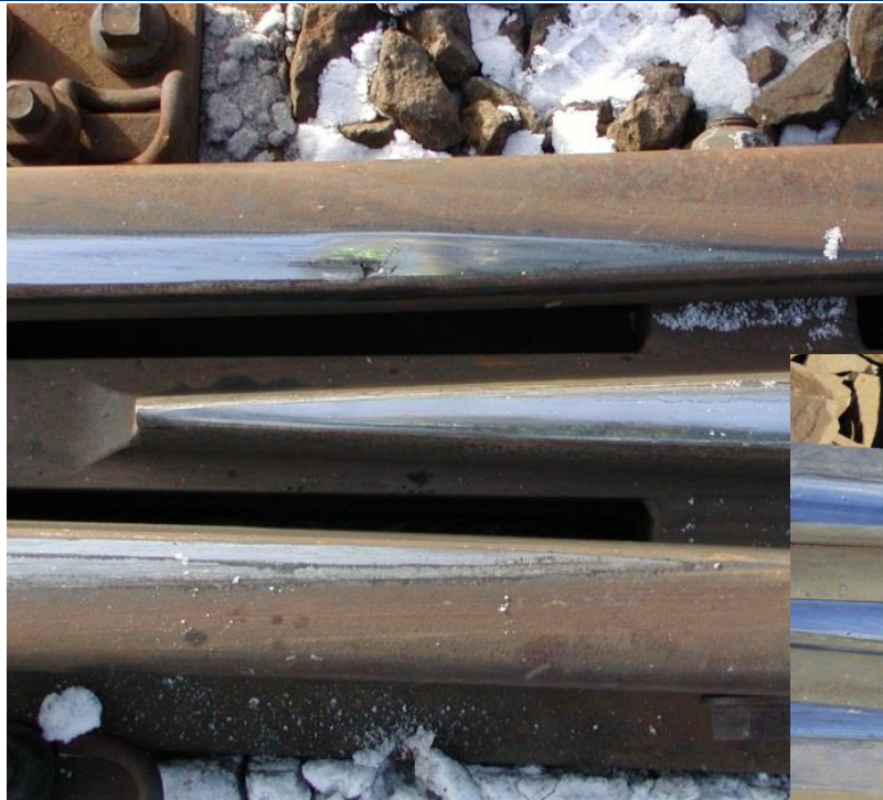
Plastic deformation of wing rails
