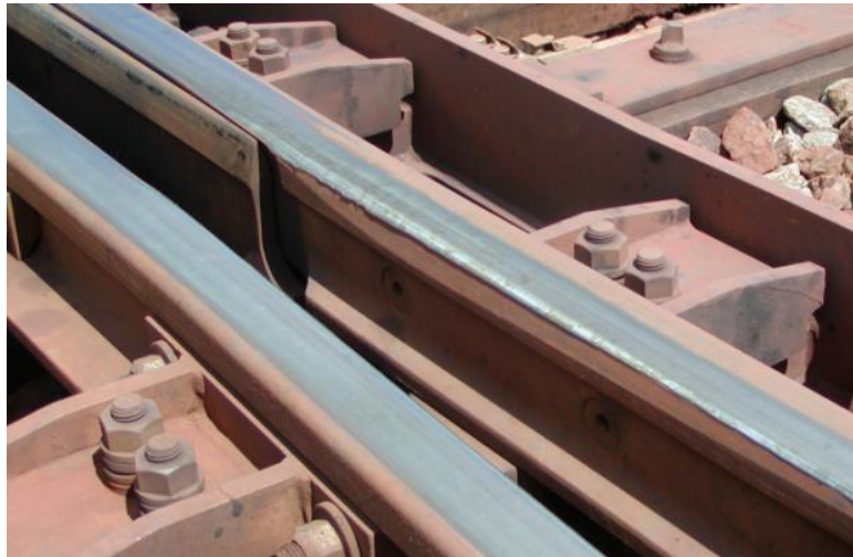
Lipping of switch/stock rails
