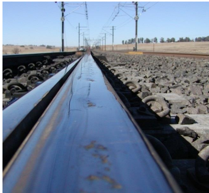
Spalling of stock rail
