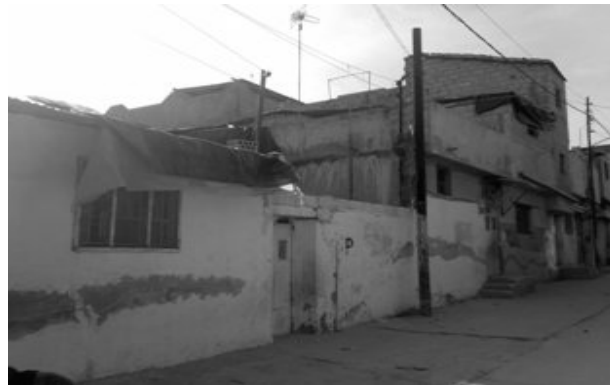
Figure 4 Plastic sheeting used for roof repairs
