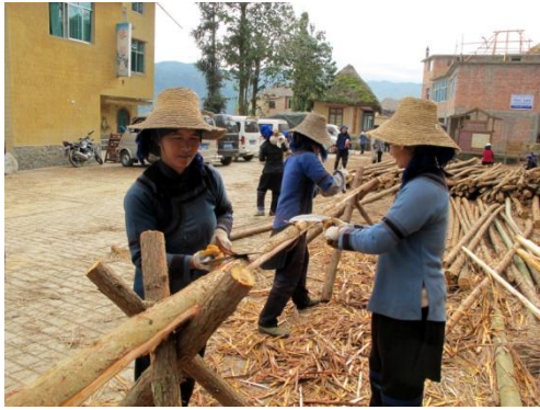
FIGURE 9. Villagers working to add thatch roofs to houses
