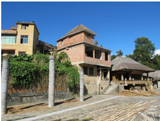
FIGURE 10. Brick and concrete houses in village in 2013
