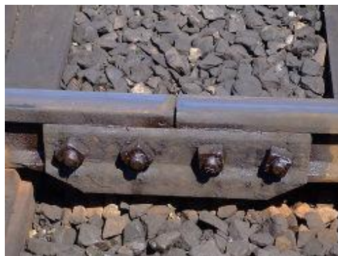
Figure 1-3 Rail joints with fishplate (Website Reference 1)
