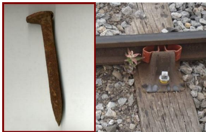
Figure 1-4 Rail spike left :( Website Reference 2) and rail chair
