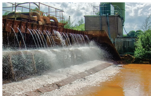
Figure 2 The weir at the treatment works, showing the transformation of colourless Fe(II)-rich minewater into orange deposits of Fe(OH) 3 (also referred to as ochre or yellow boy)
