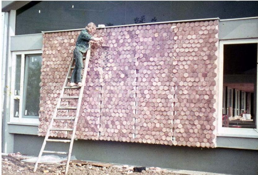
Figure D-13 Alan Martin making good the tessellation at the joints of hexagonal tiled Transform panels, unidentified European project (courtesy Fritz Steller)
