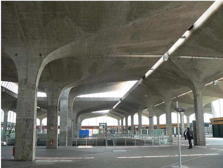
Figure D-5 RER station at Terminal 3/Roissypole, Charles-de-Gaulle Airport, Paris (2007) Arched from column to roof structure all in board-marked concrete. Down-lighters can also be seen between the units. http://fr.wikipedia.org/wiki/Fichier:Roissypole_RER_B_P1200609.jpg
