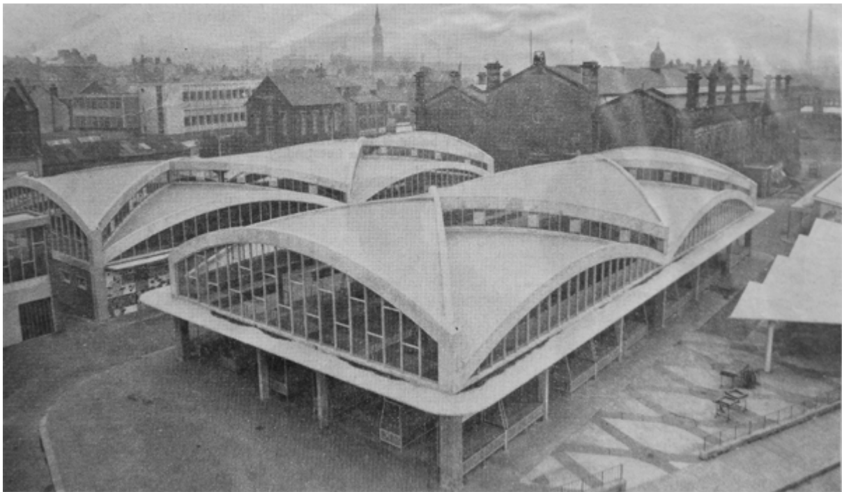
Figure A-33 Accrington Covered Market 1962. Folded plate roof over pitchers' gaffs to right (Anon, 1963g)
