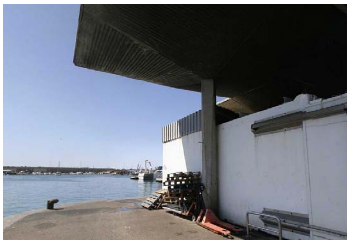
Figure 3-23 Criée Aux Poissons, Sète showing differing direction of board-marked shell soffits and chamfered columns (2011) http://www.thauenimages.fr/SETE/SETE_PORT_06.html
