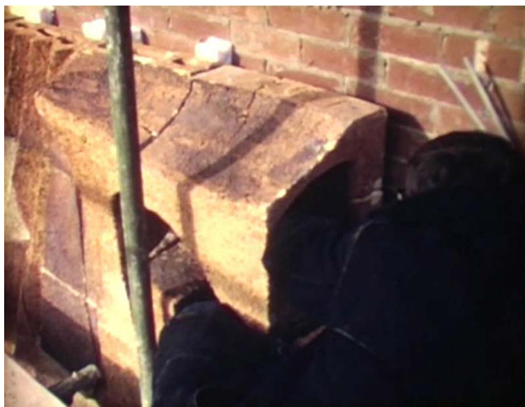
Figure 9-19 Fitting steel rods to secure a tile, from within the tile, in Huddersfield (Huddersfield Film Makers Club)
