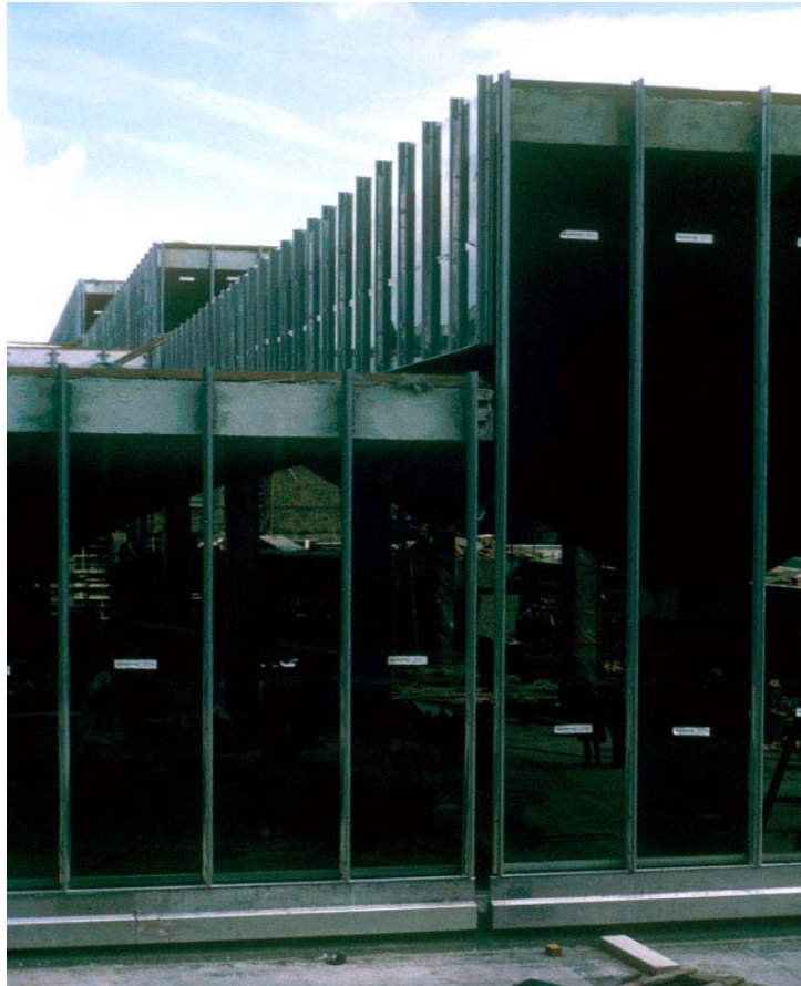
Figure 11-16 Queensgate Market. Complications of glazing showing how the change of shell is accompanied by mullions that need a membrane between (Colin Prior, 1969)
