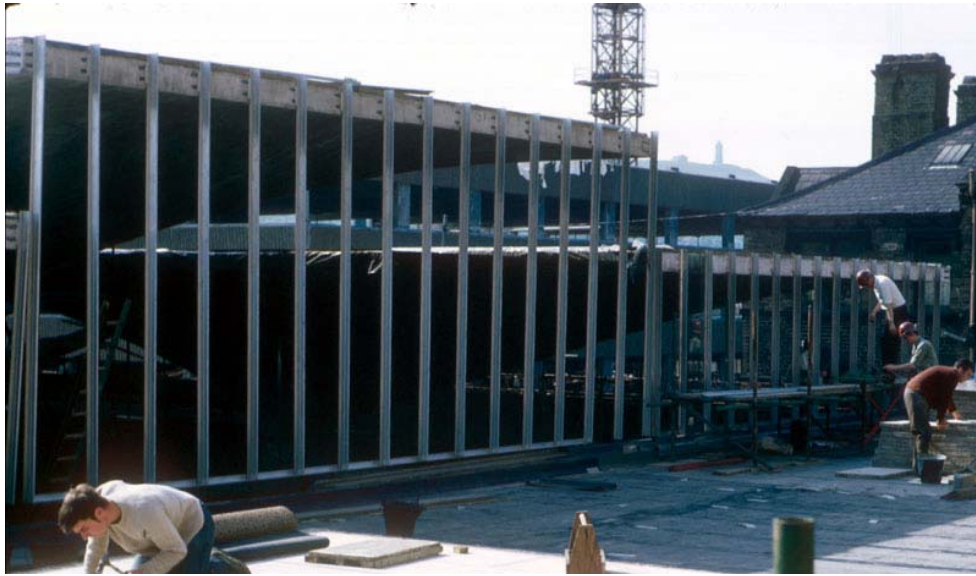
Figure 11-12 Queensgate Market. Patent glazing mullions bolted to shell perimeter (Colin Prior, 1969)
