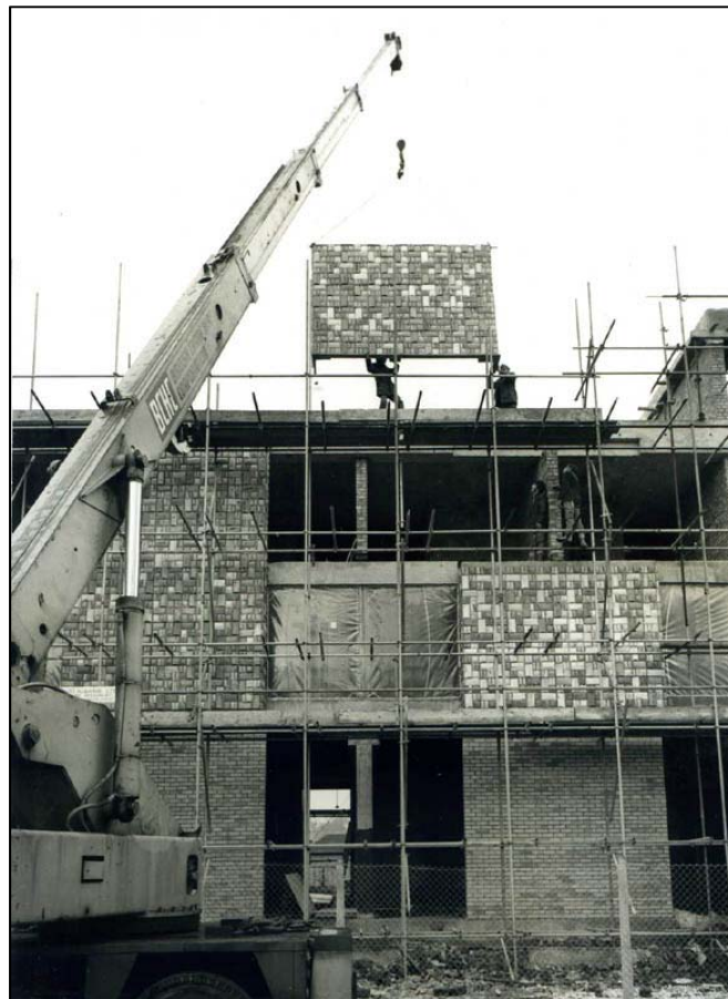
Figure D-12 Transform panel being craned onto the Luton Crest Motel, 1972. Two men on the right, mid scaffold at first floor level are waiting to receive the panel. (courtesy John Warren)
