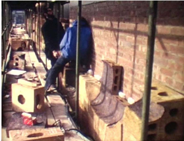
Figure 9-18 On the Huddersfield scaffold two men are manhandling a tile into position in a panel. Note packing blocks between wall and tiles (Huddersfield Film Makers Club)
