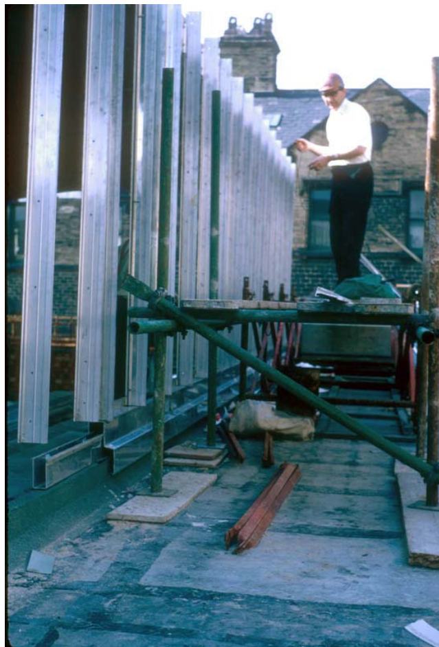
Figure 11-13 Queensgate Market. Bottom of patent glazing mullions bolted to bottom rail profile, clear and proud of U section on sill (Colin Prior, 1969)
