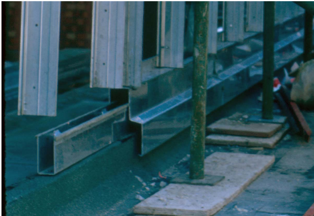
Figure 11-14 Queensgate Market. Detail of bottom of patent glazing mullions bolted to bottom rail profile, clear and proud of U section on sill (Colin Prior, 1969)
