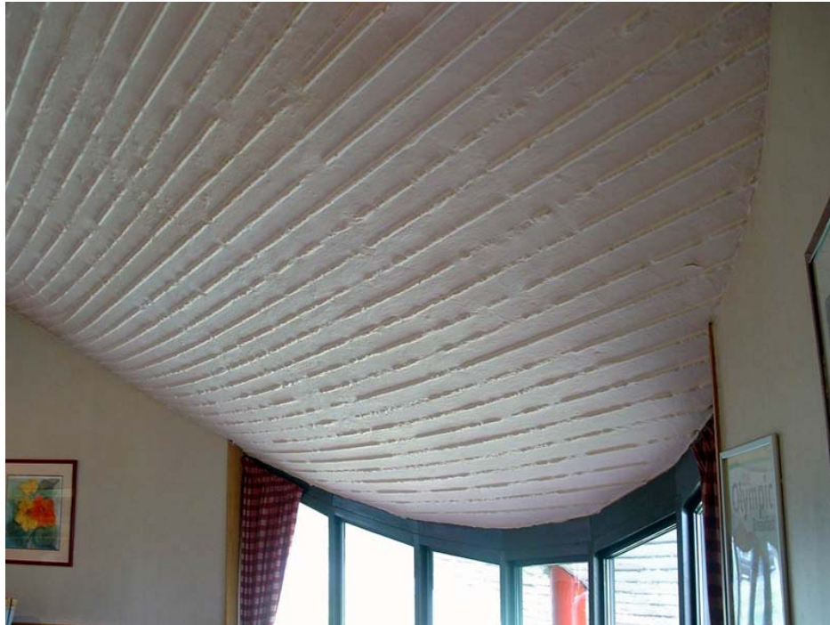
Figure D-32 Former National filling station, Markham Moor, interior showing painted shell soffit texture. (Author 2004)
