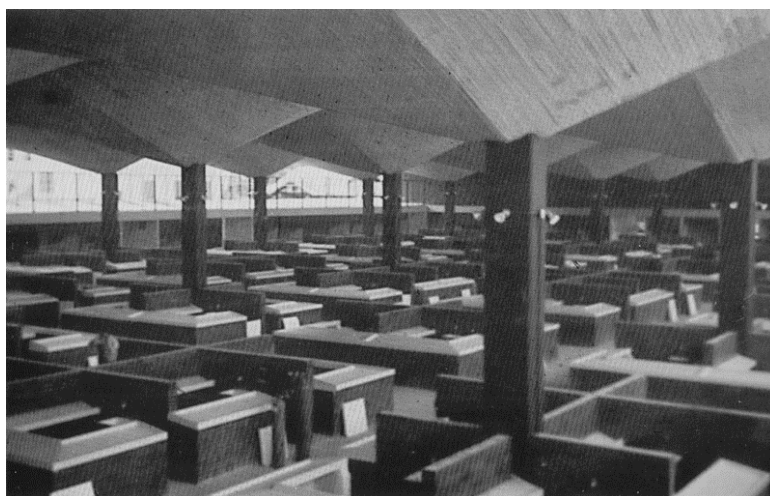
Figure 3-29 Coyoacán Market immediately after construction. Electrical conduits and down lighters are on the columns (Garlock & Billington, 2008)
