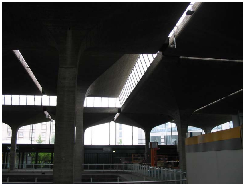
Figure D-6 RER station at Terminal 3/Roissypole, Charles-de-Gaulle Airport, Paris Bracing points and glazing mullions visible (David Shore, 2005)
