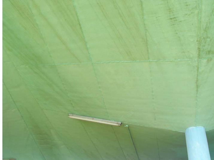
Figure 3-54 Soffit board marks and column head, Mound Stand, Gloucestershire County Cricket Ground, Bristol (Author, 2012)
