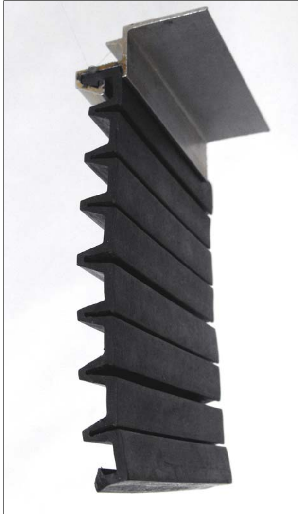
Figure 11-9 A manufacturer's 105 x 80mm sample of the EDPM concertina membrane with a Heywood Helliwell aluminium profile from the 1968 design process of Queensgate Market's glazing (Author, 2012)
