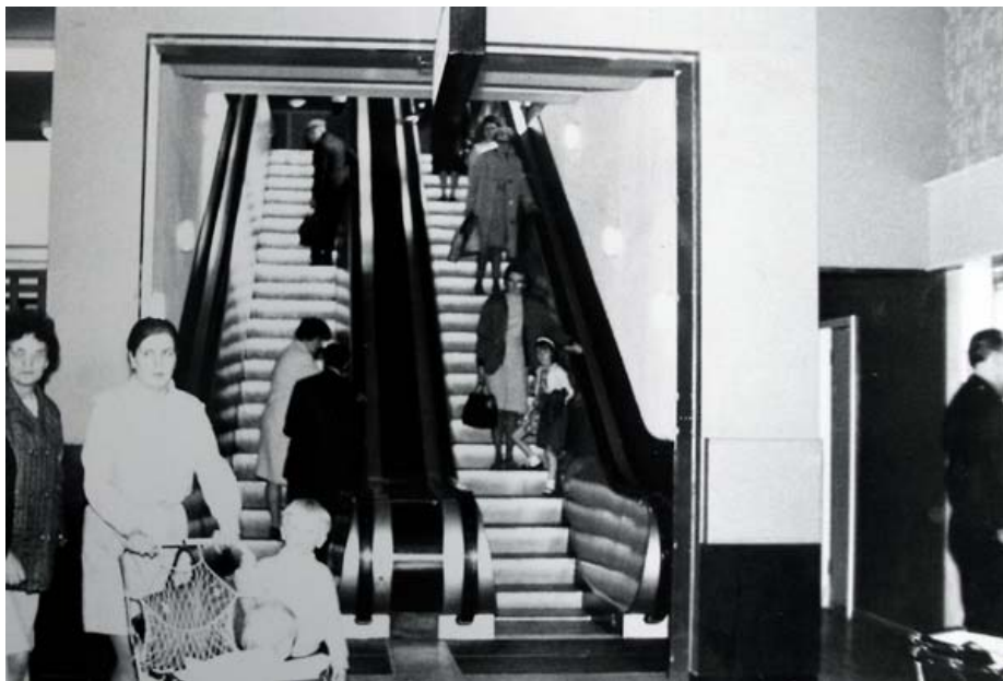
Figure 6-41 Nelson Market Hall, escalators to and from the Arndale Centre above. Abstract relief pattern tiles top right (1967- probably 1968). Source Nelson Library The hall has massive rectangular concrete columns, at 36' centres, supporting the centre above. Columns in the aisles were clad with Formica like framed panels to the height of the stall fascias (Figures 6-42 & 6-43). A wall was clad with abstract relief tiles (Figure 6-41 and Figure 7-21) (discussed in chapter 7).
