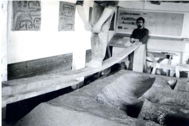
Figure 9-11 Alan Martin pulling cutting wire through an Articulation in movement panel, Frank Maurier looking on. Note large maquettes and copies of the architect's Market hall elevation drawings on the walls (John Warren)
