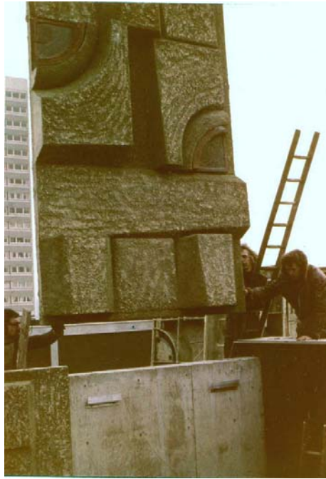
Figure D-8 Panel unit being craned in to position at Castle Vale
