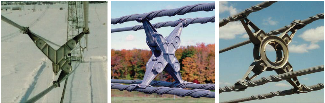
Figure 1: Spacers in triple and quad bundles
