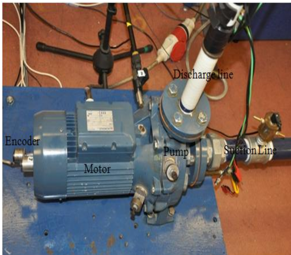
Figure 3.2. The test-rig pump.
