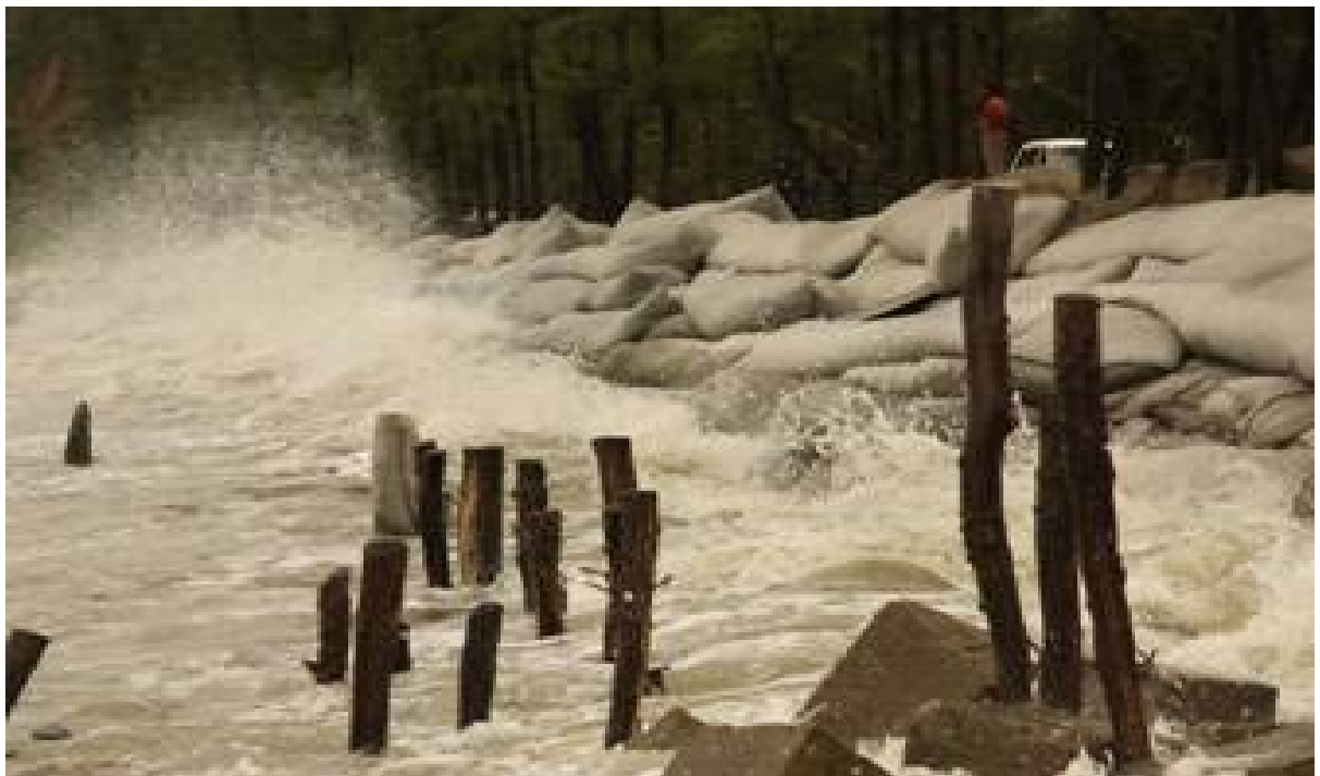
Figure 6.12: Protection of marine drive from strong tidal surges.
