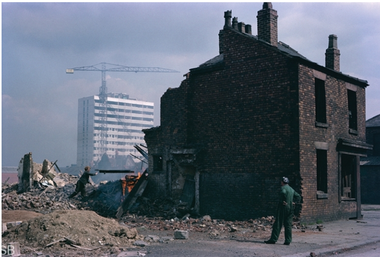
Figure 1: Demolition in the shadow of new development, Shirley Baker
