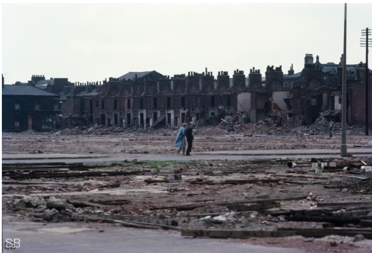
Figure 2: Partial demolition in Salford clearance area, Shirley Baker
