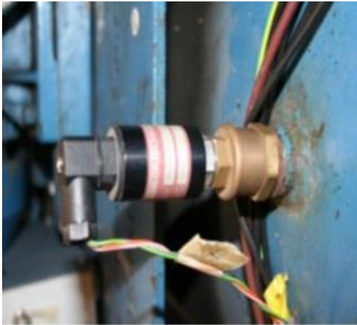
Figure 4-7 Static pressure sensor on air storage tank
