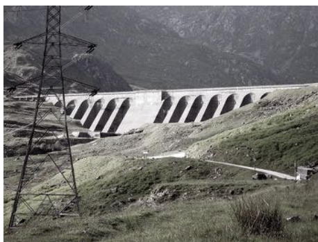
fig. 2.11 - The Cruachan Power station. Performances happen one mile underneath.
