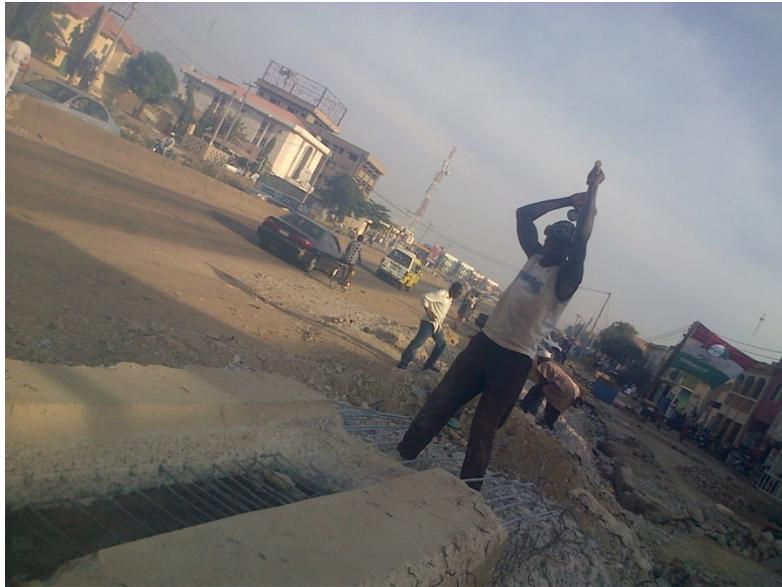
**Figure 33: Self-employed *Dangwangwan* breaking concrete to salvage reinforcements for sale**
