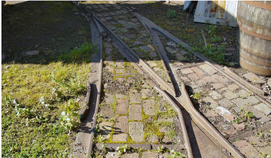
1803, Plateway for cylindrical wheels
