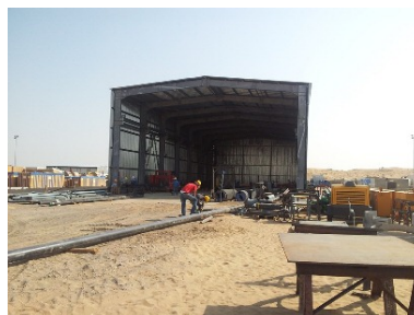
Figure 2: Pipe Spool Prefabrication Workshop
