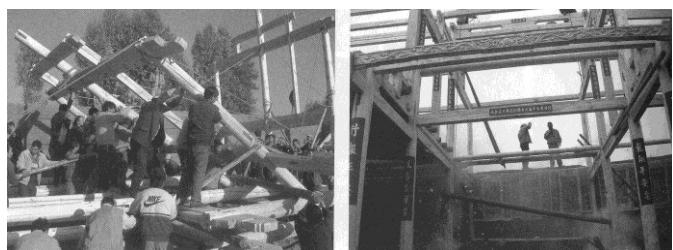
Figure 33: Erecting the timber framework and sticking couplings on the beams and columns (Bin, 2011, p.132)
