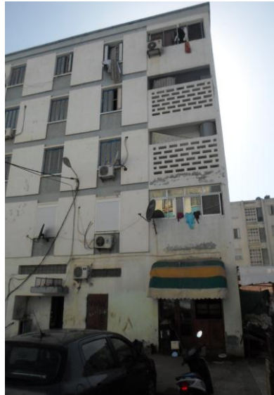
Figure 3: Example of ‘closed’ balconies
