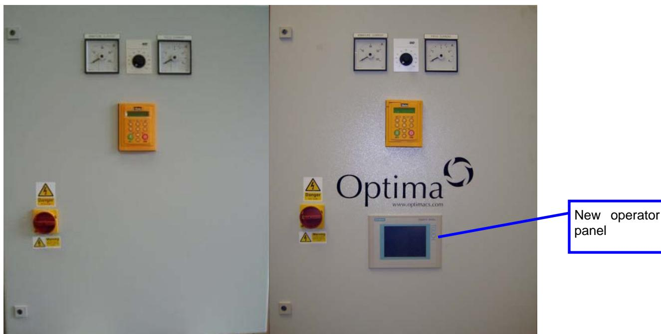
Figure B-2 - Test rig panel exterior before and after modification
