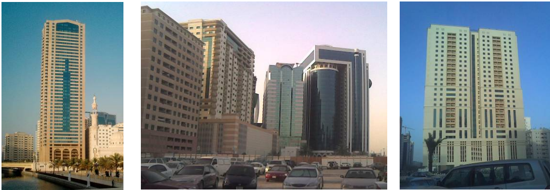
Figure 6.10 – High-rise residential buildings in Sharjah - UAE
