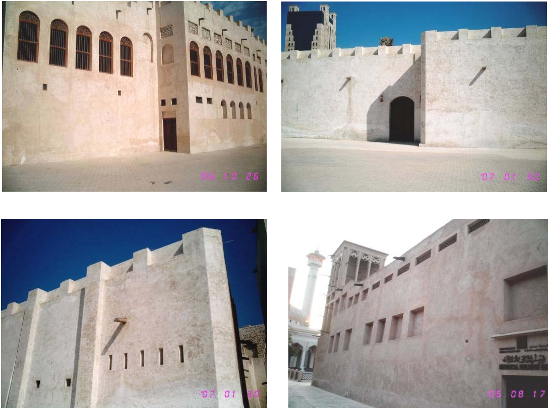
Figure 6.27- Solid elevation with small openings to keep privacy of the indoor spaces
