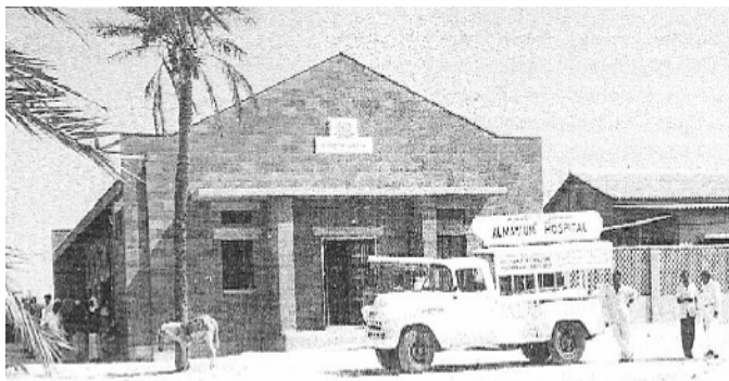
Al Maktoum Hospital in Dubai (Source: Dyck, 2004)
