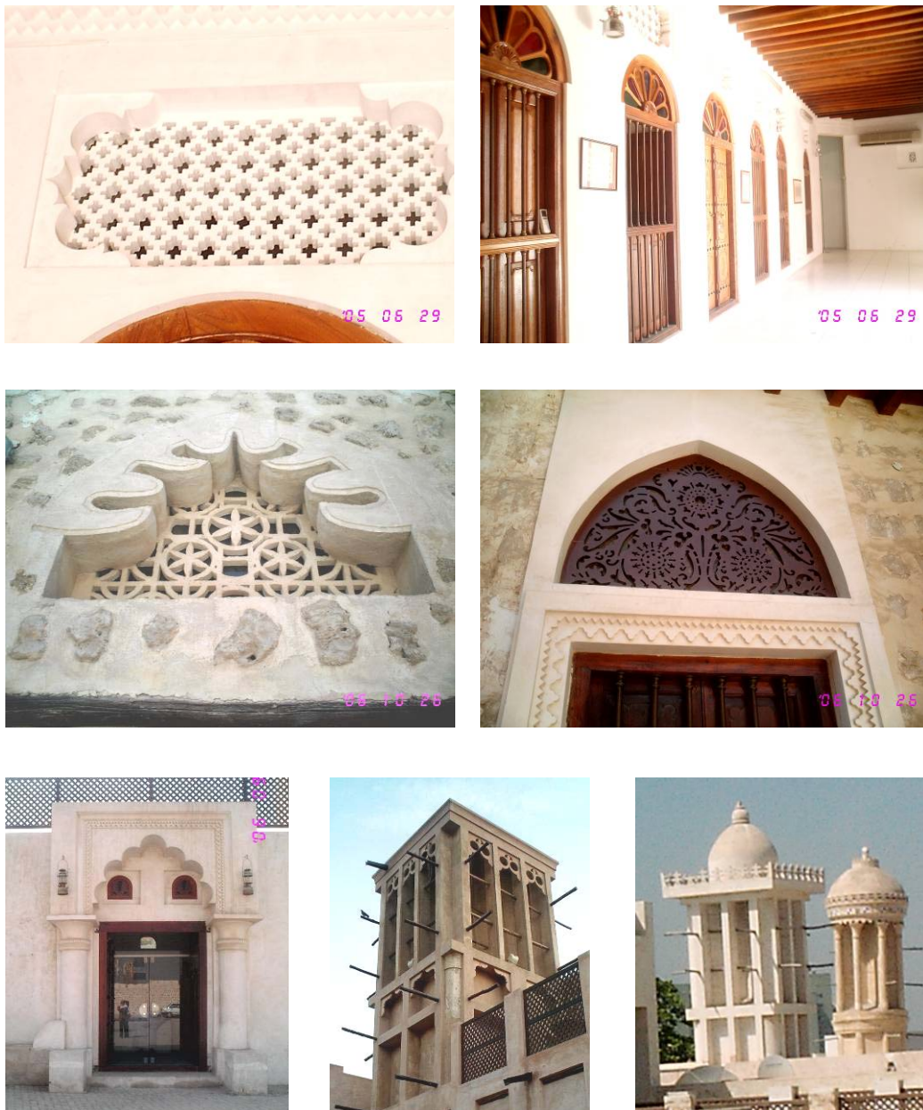
Figure 6.34– Decoration are added for different features in traditional houses in the UAE
