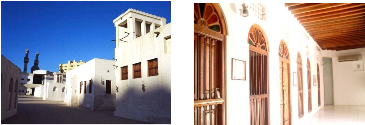
Figure 3.32 -Restored traditional buildings in Sharjah
