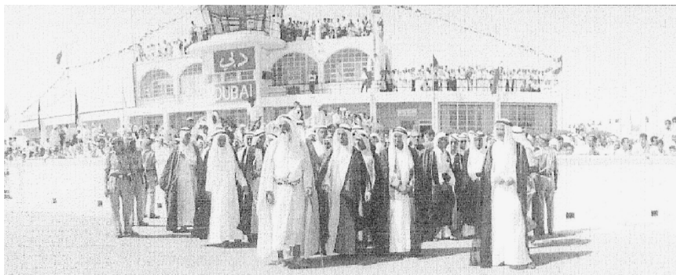
Figure 3.19- Dubai airport in the 1960s
