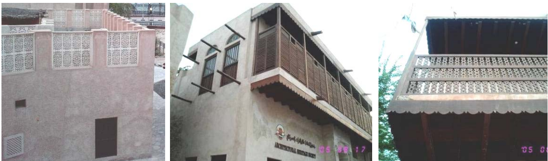
Figure 6.28- Balconies, projections, and parapets were well screened to keep privacy
