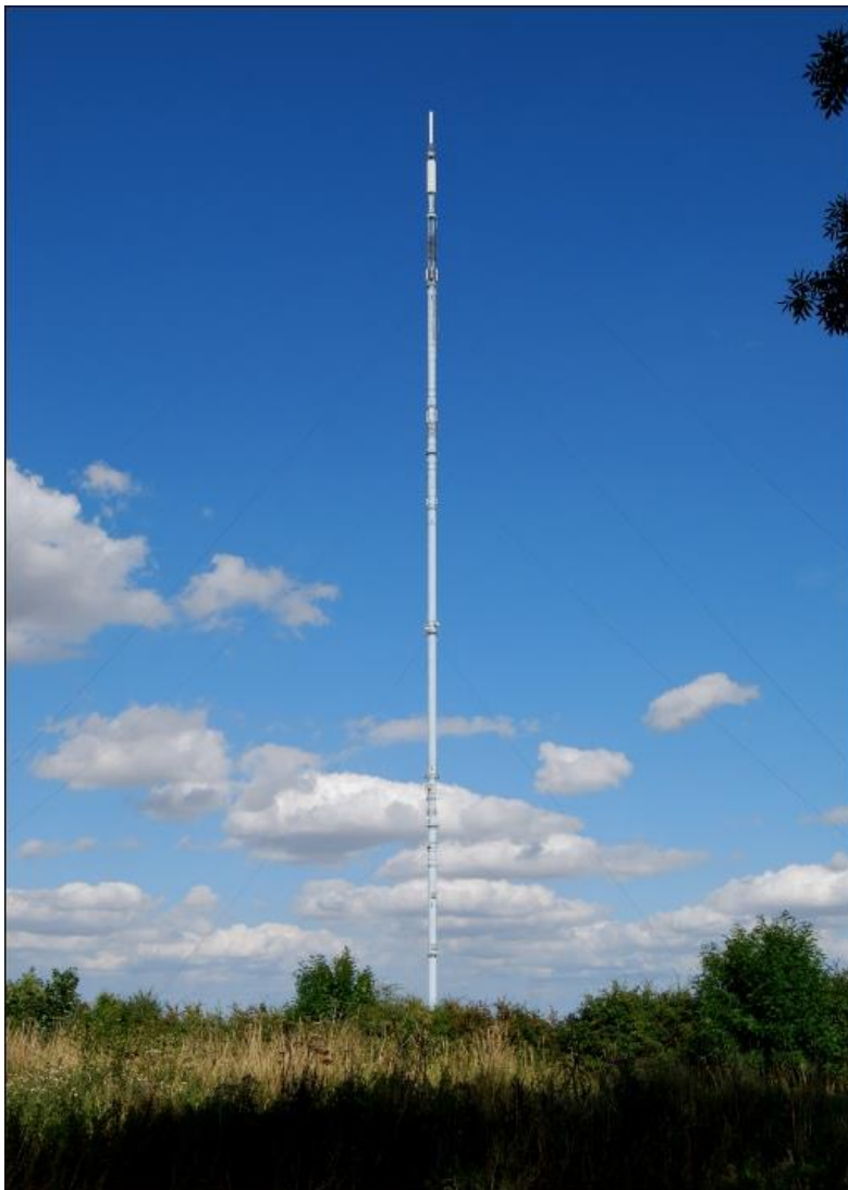
Figure 67. Belmont transmitting station.
