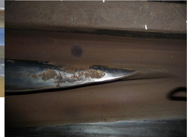
Spalling & plastic deformation of crossing nose
