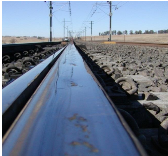
Spalling of stock rail
