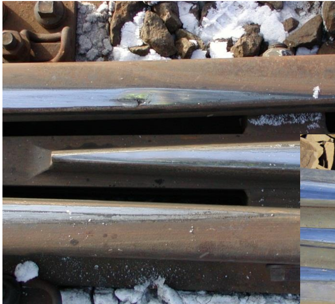
Plastic deformation of wing rails
