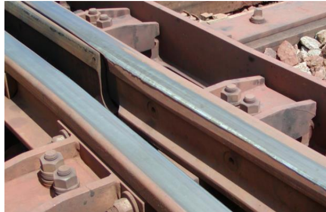
Lipping of switch/stock rails
