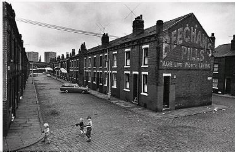
Figure 1. Terraced Housing built in the 1900's shown in the 1960's 3
