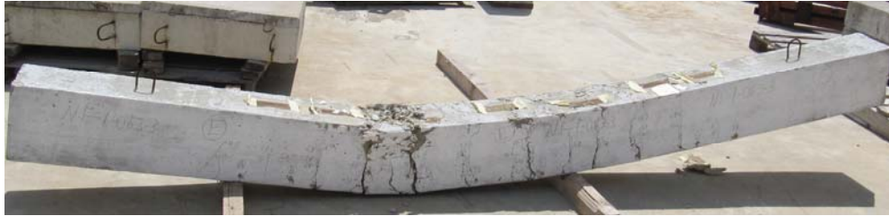
(a) The damaged beam
