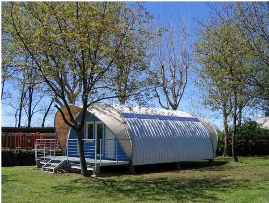
Figure 4 – L’Armadillo housing unit in Carate Brianza (Milano) integrating photovoltaic cells on the roof.
