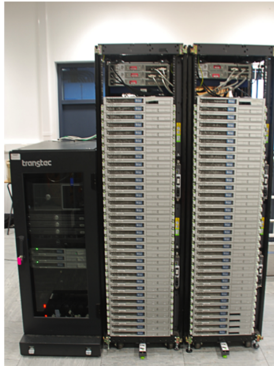
FIGURE 5.3: SOL Cluster in the University Datacentre
