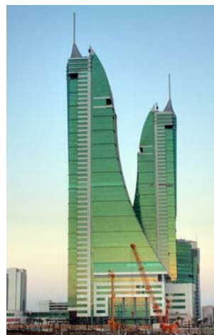
Dino-architecture? Bahrain's twin towers are covered in glass. Allan Donque, CC BY
