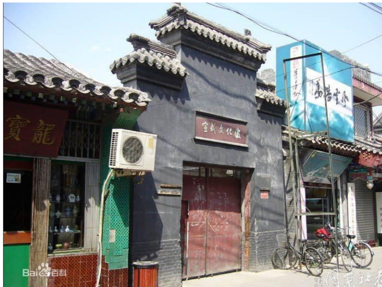
Fig 3.4: External electric wires and air-conditioners
