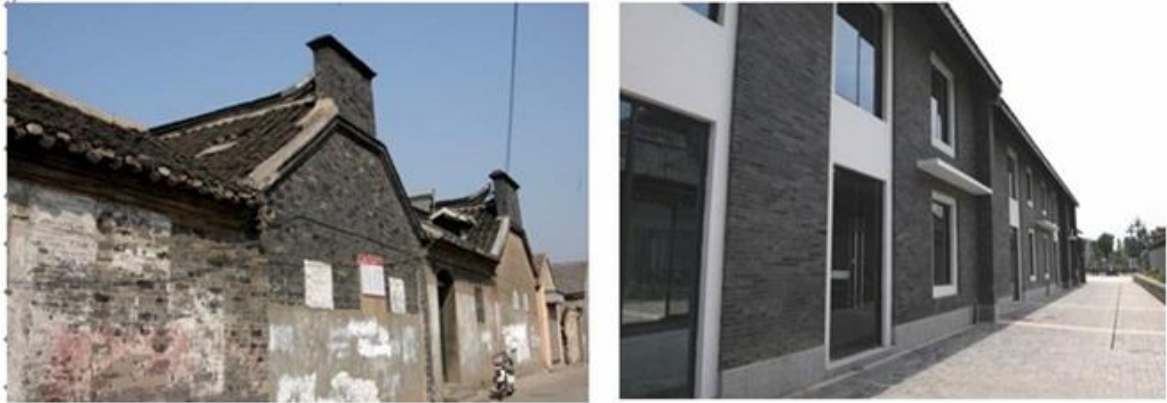
Fig 6.13: The houses before and after Fashion Island was built
