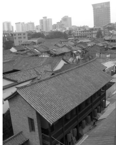
Fig. 1. Traditional and modern buildings in Kunming
