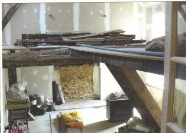
Watching a project taking shape is very satisfying
