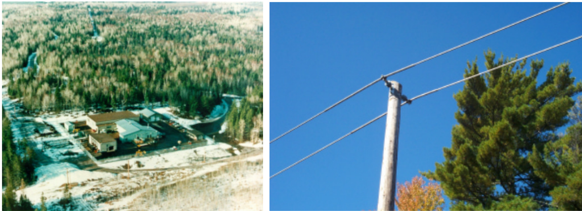
Figure 2.3: Wisconsin ELF transmitter site (Left), view (right) of a typical ELF antenna [23]
