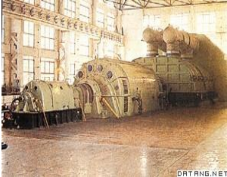
The steam turbine generator set
