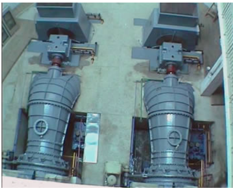
The hydroelectric generator set
