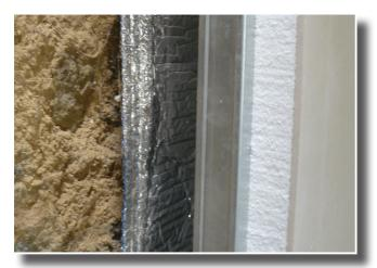
(10mm plasterboard with 40mm of foam). The walls had a similar quilt liner, followed by an aluminium frame and the same insulated plasterboard.
