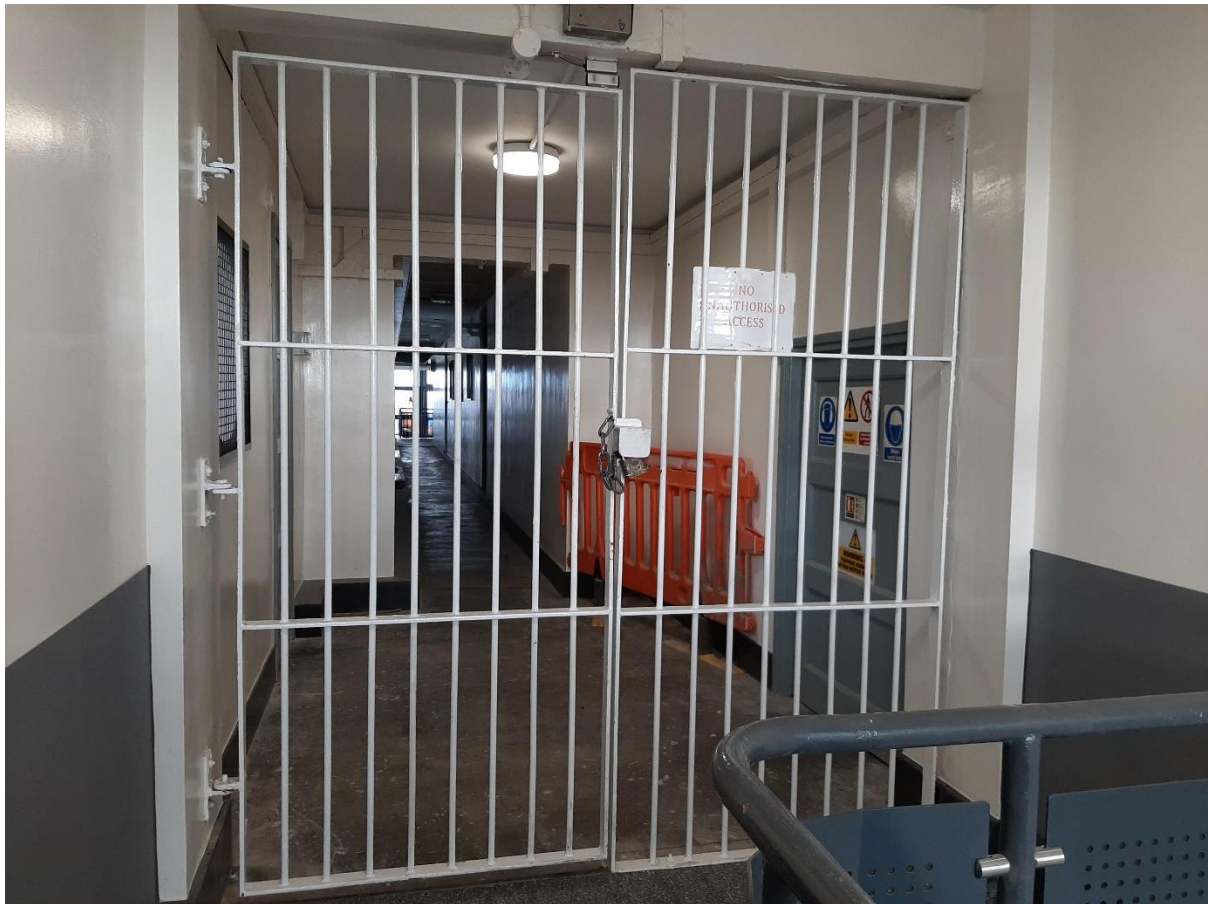
Figure 6: Gated-off connecting corridor on the twelfth storey of each CSS tower block. These gates were installed during the 1989-1992 refurbishment at the request of the Four Towers Tenants' Association to prevent use of the connecting corridors by anti-social elements. They are unlocked by the caretakers when one of the lifts on either side of the block breaks down. And do not compromise fire safety, because each side of the block incorporates compartmentation with its own staircase, lift and access to the unique emergency fire-escape staircases that serve each flat.
