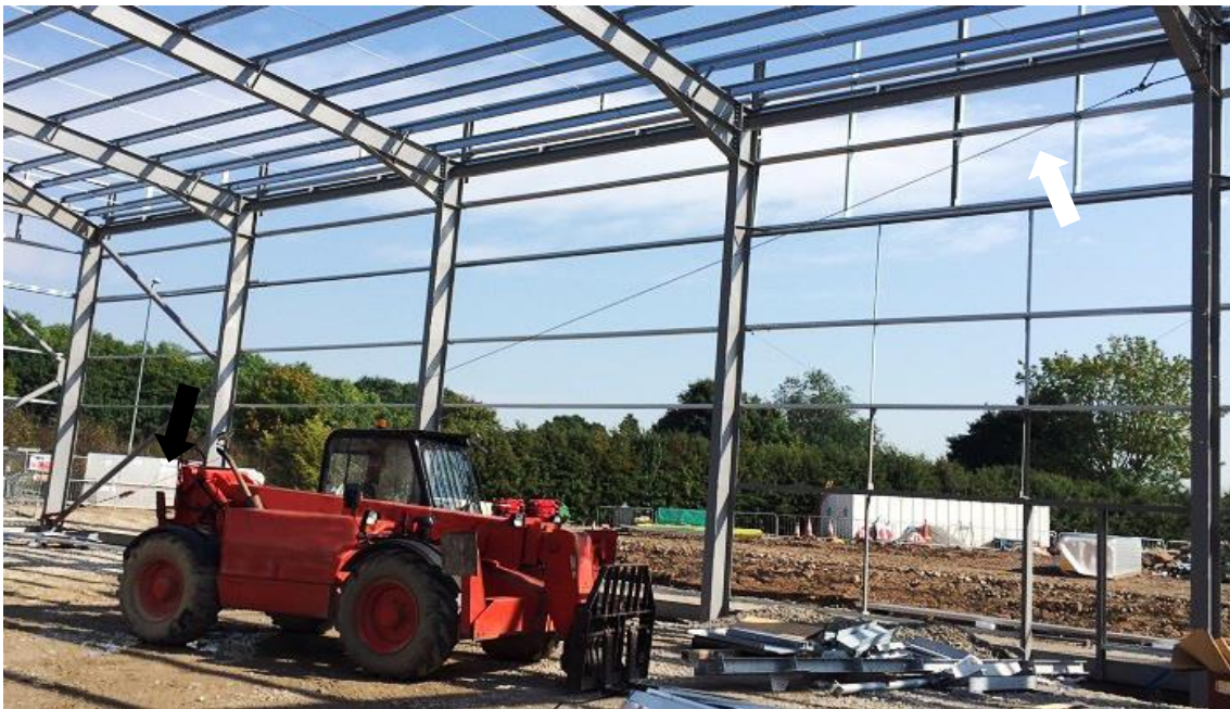
Figure 4-49. A portable manual hoist along with maxiflex wire rope being used to pull the steel frame to an acceptable position and orientation
