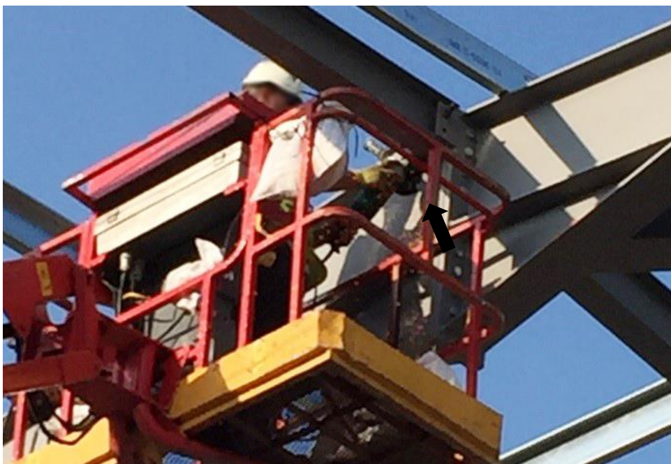
Figure 4-51. The steel erector trimmed the beam
