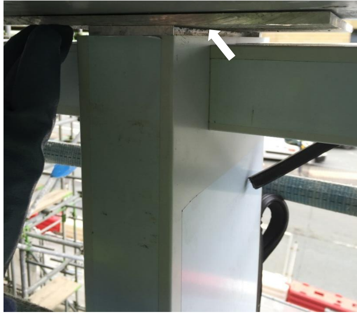
Figure 4-16. Adjustable connections for curtain walling
