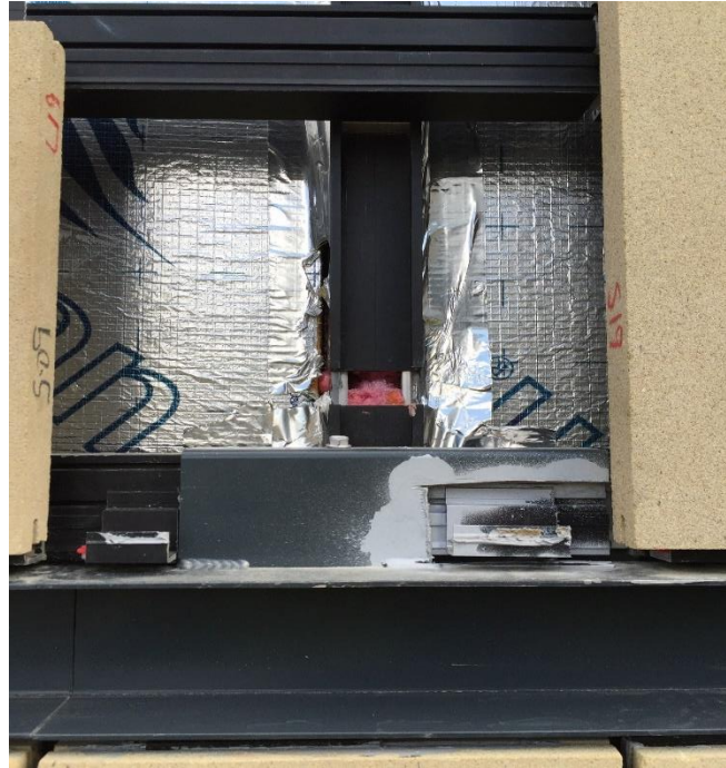
Figure 4-13. Expansion connection for stone cladding
