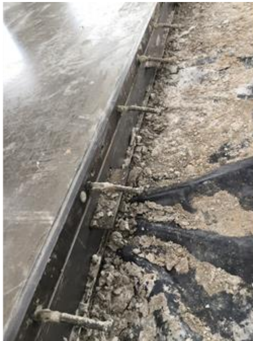
Figure 4-26. Butt connections for the interior concrete slabs
