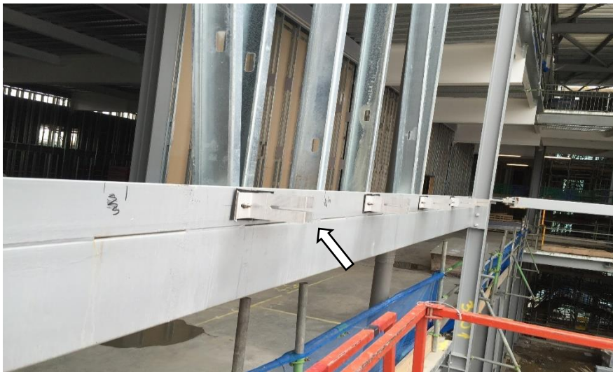
Figure 4-15. Cladding brackets and their slotted heads
