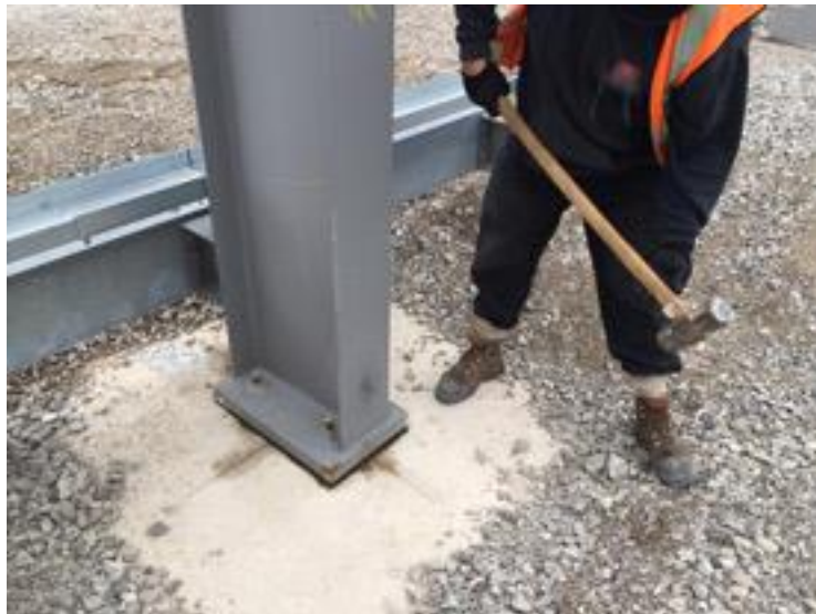
Figure 4-29. Moving the columns using a hammer
