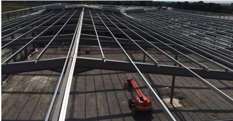
Figure 4-37. Installed purlins on the roof
