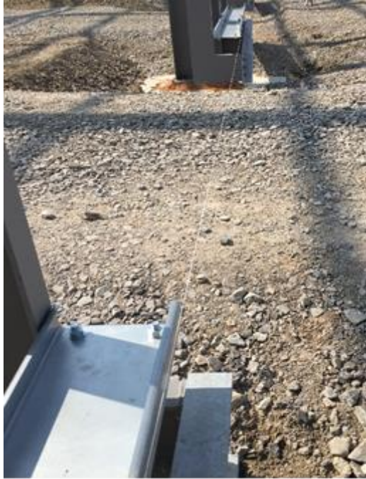
Figure 4-33. Use of the string to control the alignment of doorways
