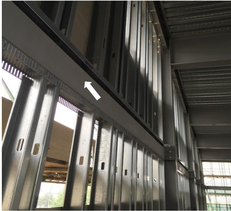
Figure 4-14. Slotted head track in exterior walling system
