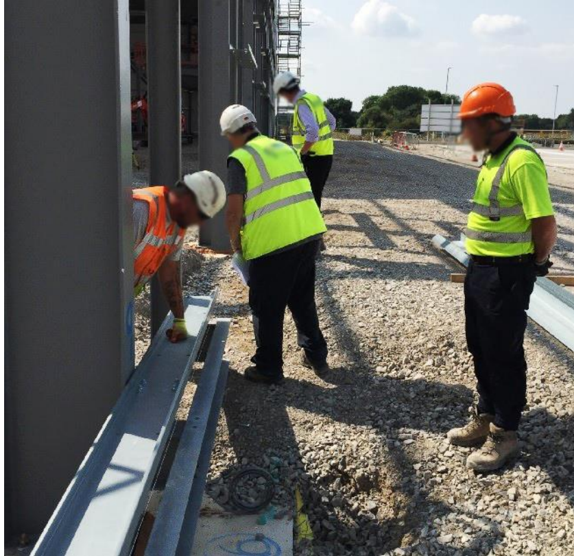
Figure 4-32. Staff involved to solve the problem with doorways
