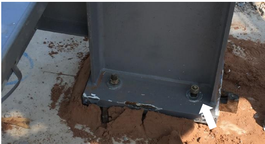
Figure 4-35. Bolts are loosened at the front to adjust the columns in the desired orientation
