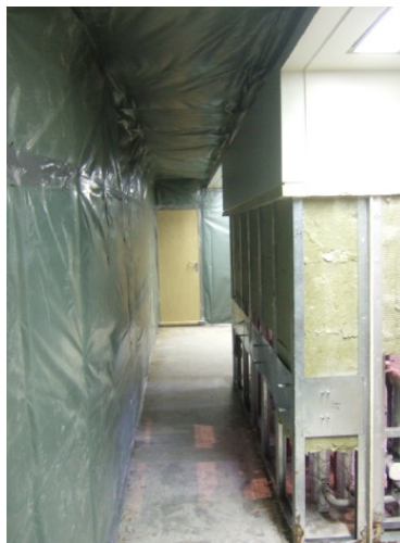
Figure 4 - Dust protection - view from a renovation area (Ross et al., 2011)
