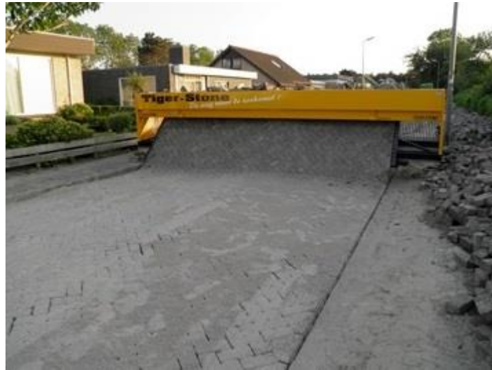
Figure 18: A concrete paving robot in the Netherlands (Tiger-Stone, 2015)
