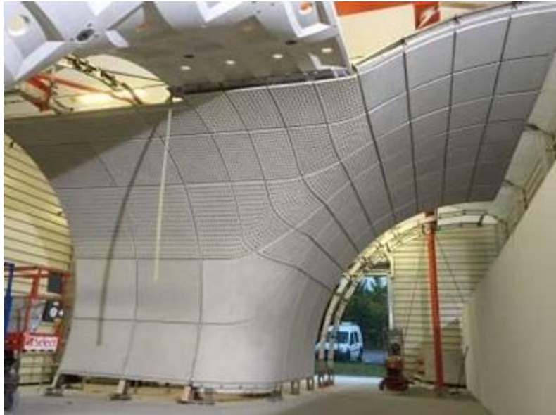
Figure 14: Complex-shaped glass reinforced linings (cladding) that were manufactured using the 3D mould printing technology
