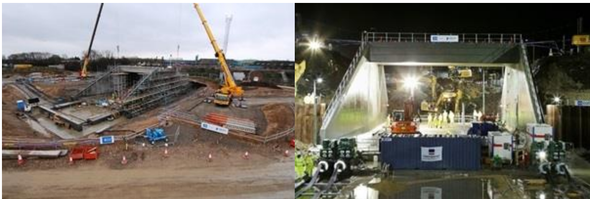
Figure 23: A 4000 tonne bridge was slid in its place on a bentonite bed in 76 hours within the A160/A180 Port of Immingham scheme using hydraulic jacks during the Christmas holiday in 2015 (Department for Transport, 2015)
