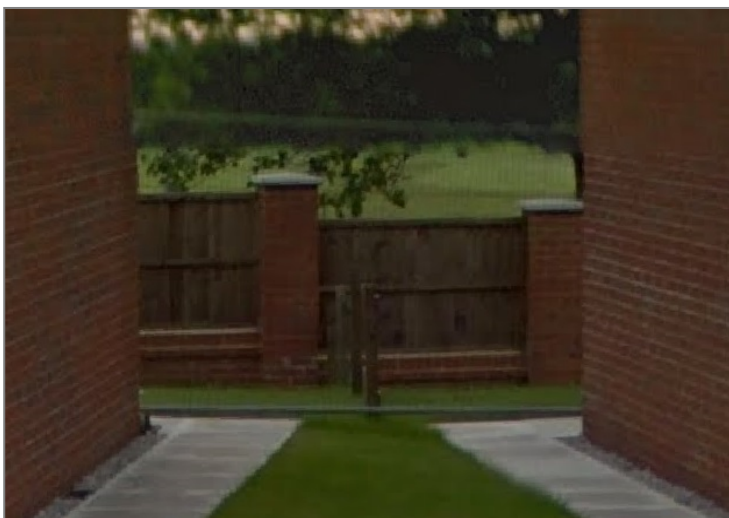
Figure 34 Rear boundary at CIS-2
