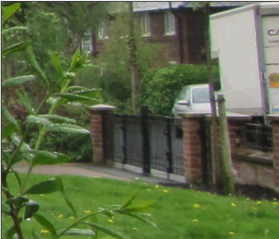
Figure 39 Defensible space to the front of the development
