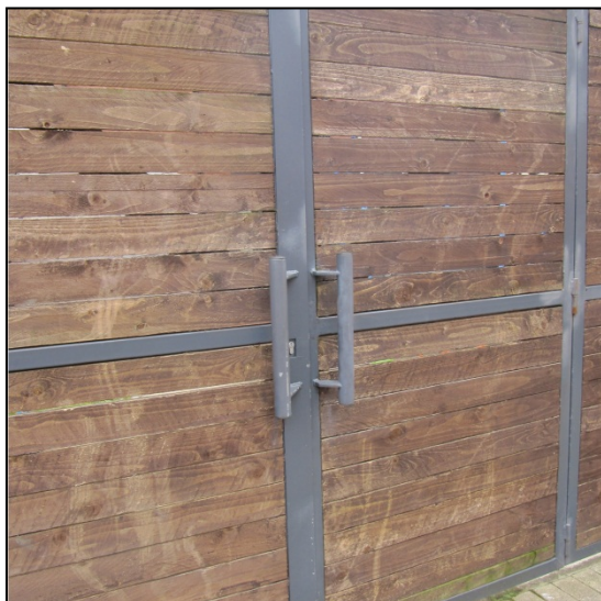
Figure 23 Doors installed to secure in-curtilage car parking space
