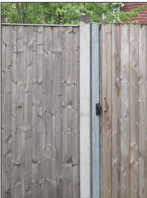
Figure 40 Slam-to-lock on a side gate
